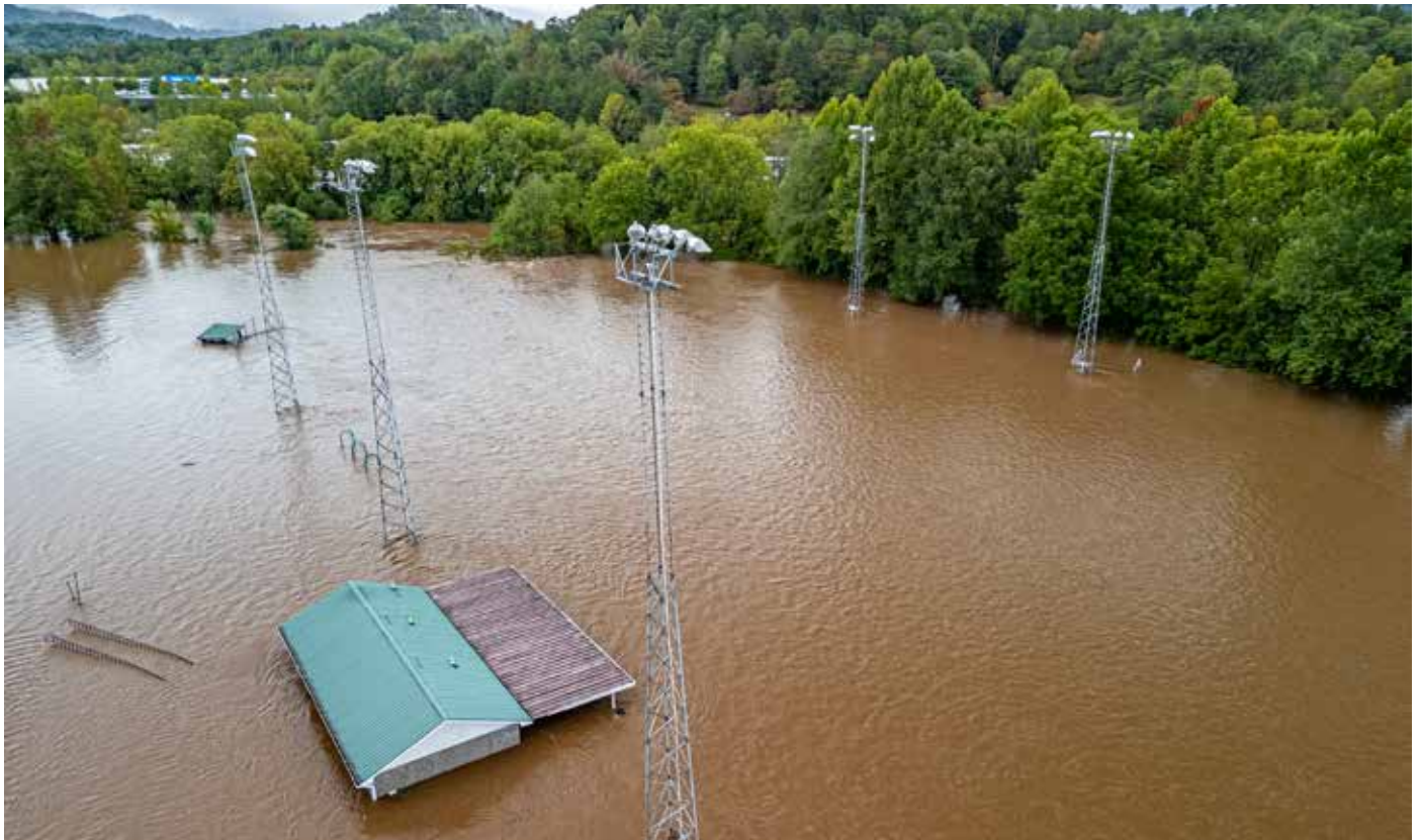
Hurricane Helene causes flooding in Western North Carolina.
